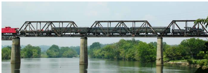
The Three Rivers Trestle
